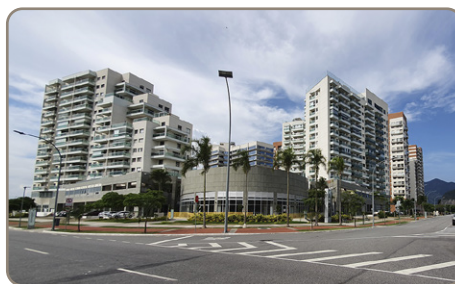
UNION SQUARE (MALL E WORK)
